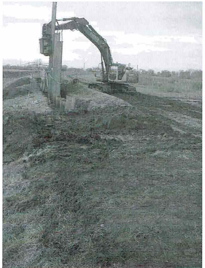
Piling works using Movax hammer and excavator, Marsh Drain, November 2014
