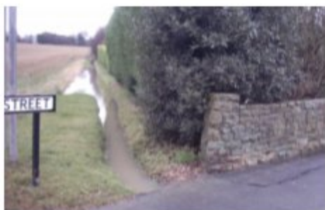
Day after flood water on road – can be much worse than this
